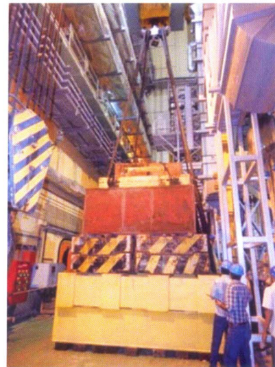
Figure 9. 280 tons Load being lifted during full load test.
