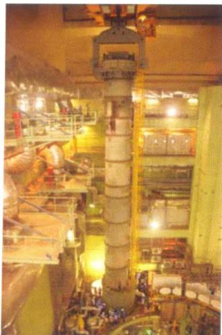
Figure 11. PI Flask (230 tons) lifted inside RCB.
