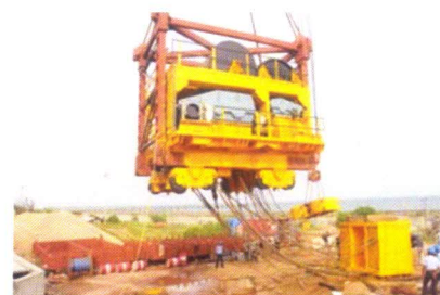
Figure 5. Trolley assembly being lifted with the hooks.
